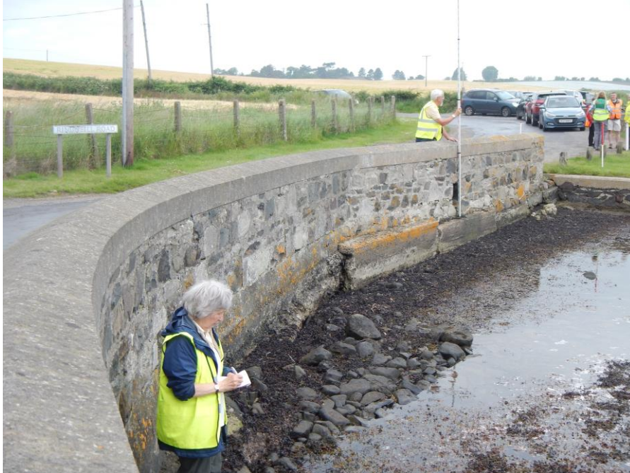
Figure 08: View of south-western sea wall, looking west
