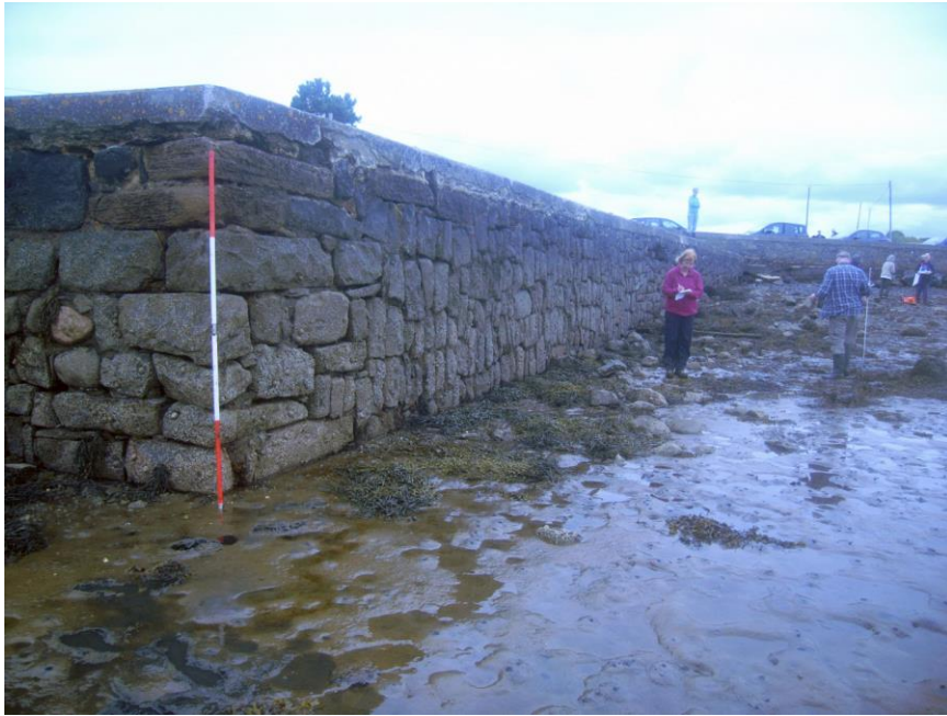
Figure 10: View of north-facing wall of quay, looking west
