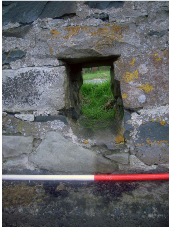
Figure 18: Mooring point re-used as drainage channel
