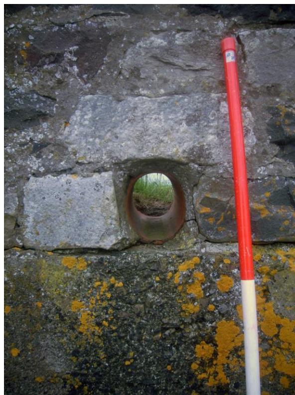
Figure 19: Mooring point re-used as drainage channel
