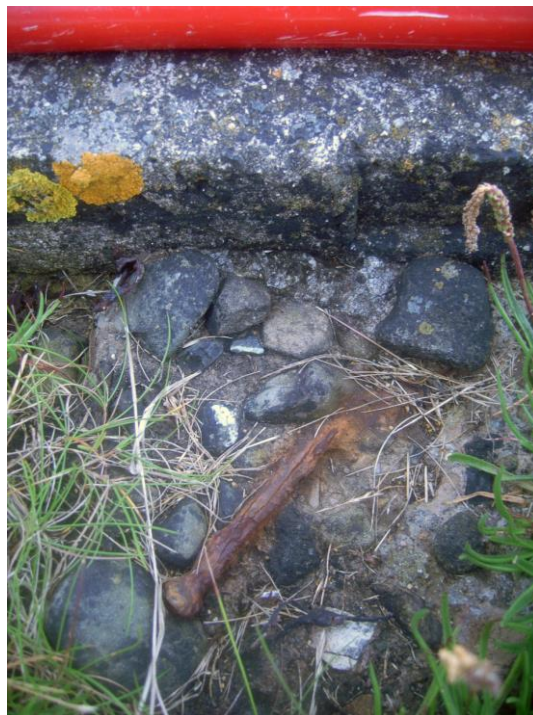
Figure 11: Quay composition materials, including iron nail
