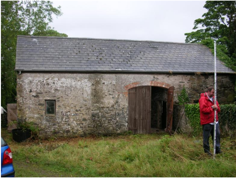
1. Creamery looking to the north east
