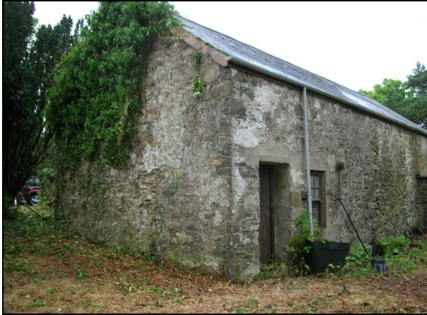
Figure 24: Creamery looking to the west
