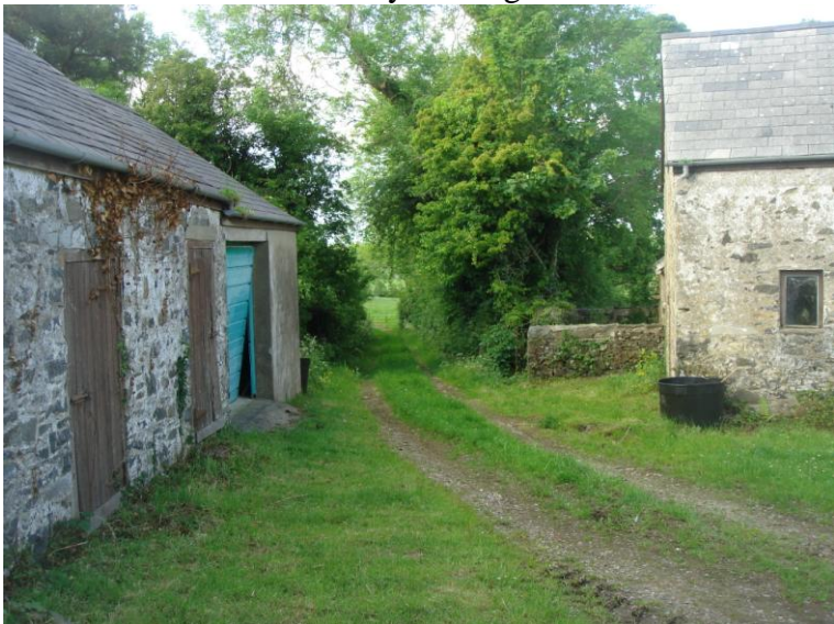
5. Store/garage looking to the north
