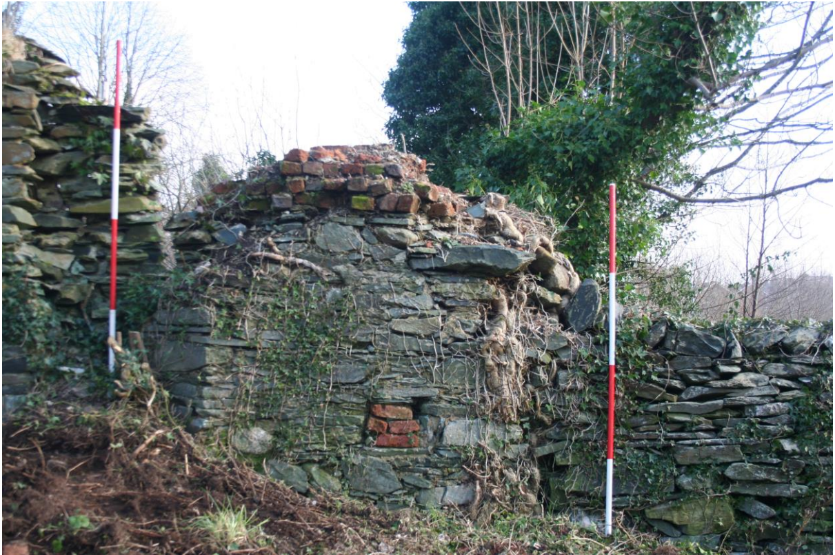
Photo 1: Section of curving masonry from south prior to the excavations showing brick blocked gun loop
