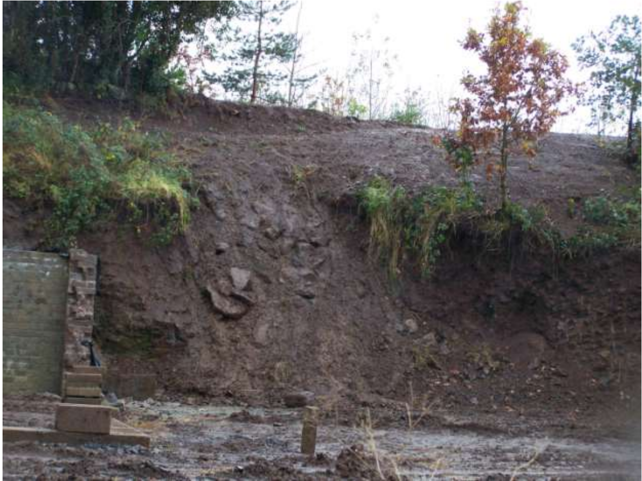
Photo 5: Souterrain backfilled at the end of the excavation.
