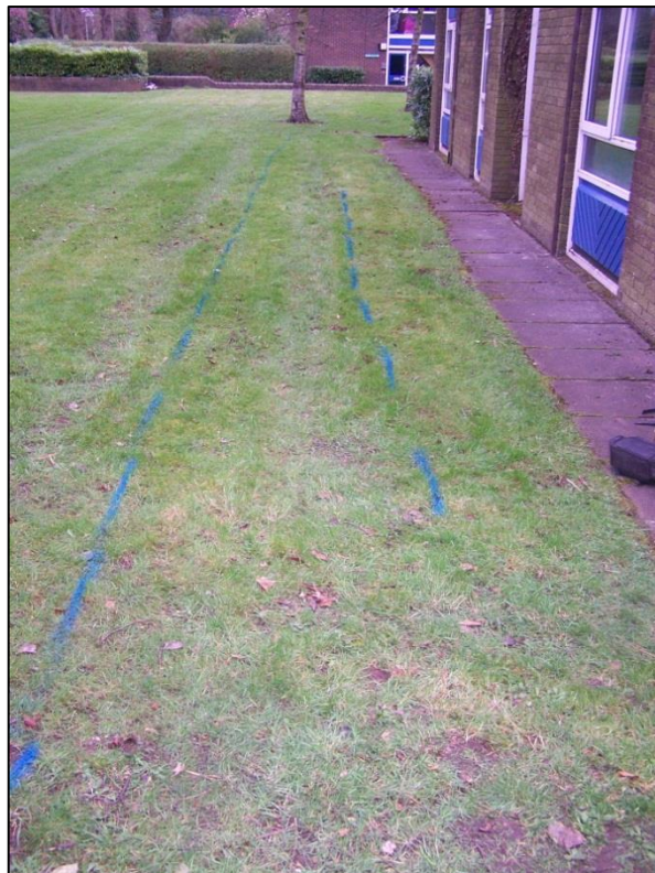
Plate 6: Trench 2 prior to excavation looking west
