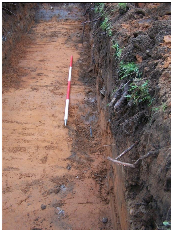
Plate 12: Cable trench (307 & 308) in trench 3 looking north
