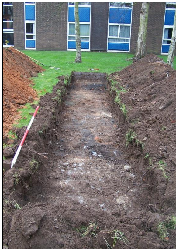
Plate 14: Post-excitation photo of trench 4 looking north
