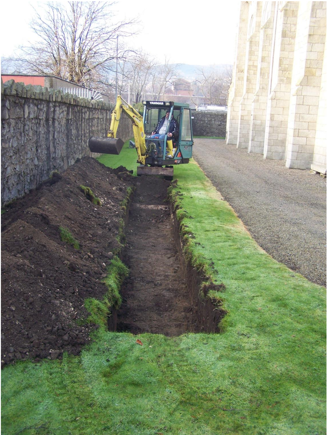
Plate 2: Excavation of Trench 1, looking west.
