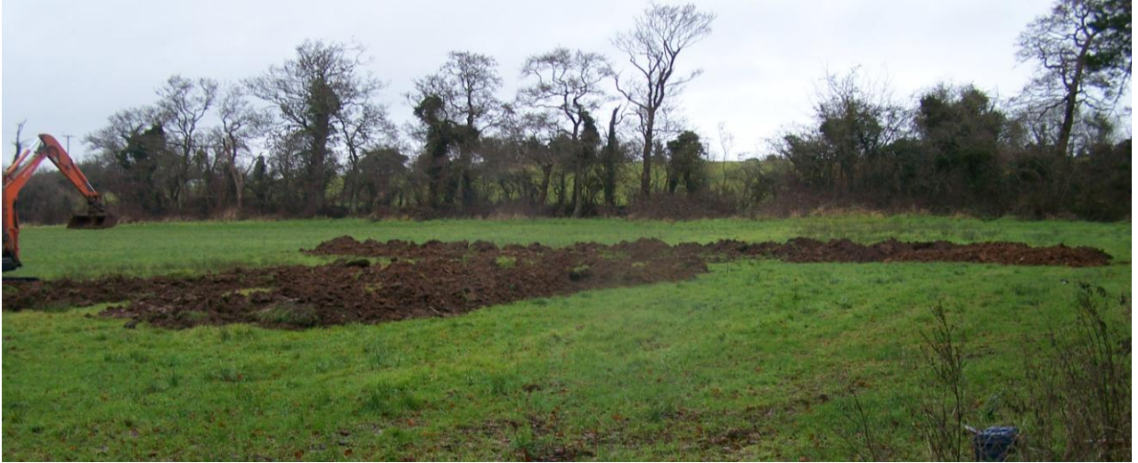
Plate 1. The five excavated test trenches. From the south.
