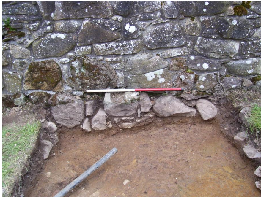
Plate 2: Close-up photograph showing eastern bawn wall foundation (context 106) built directly upon subsoil in Trench 1
