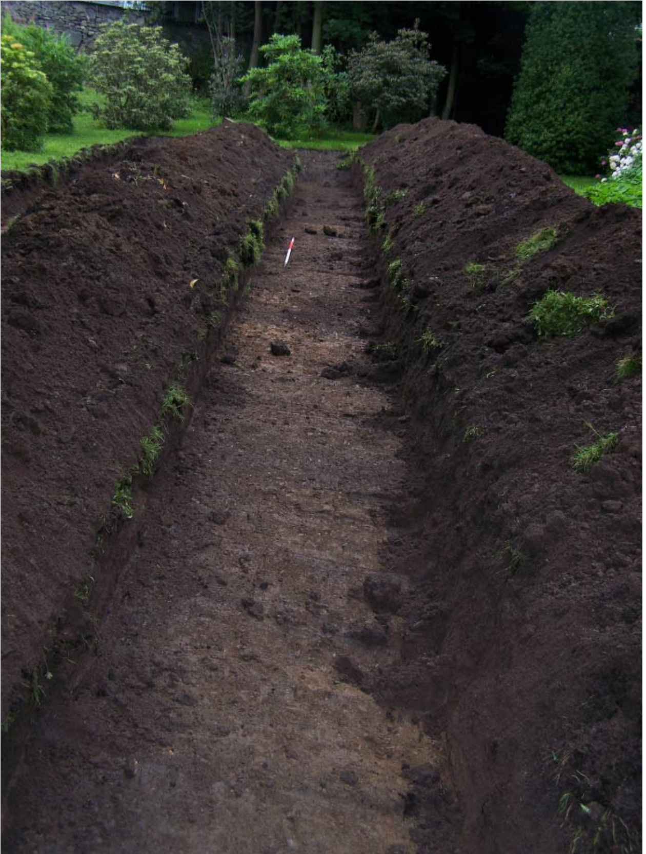
Plate Seven: Trench Two following excavation to subsoil level, looking north-west
