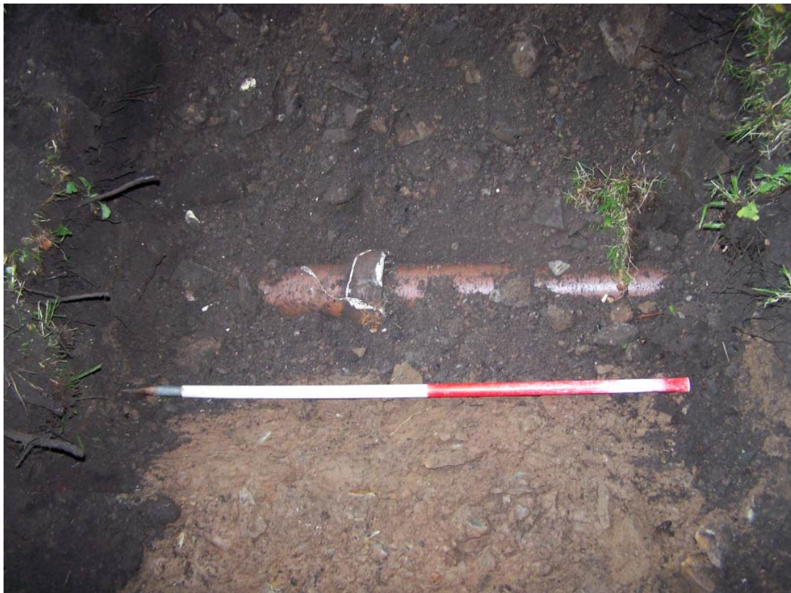
Plate Five: Cut of sewer pipe (Context No. 103), looking south-east
