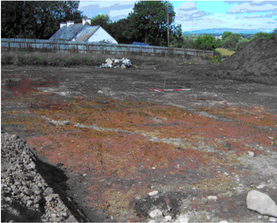
Plate 8 View of development site excavated to glacial subsoil level, showing dark staining of subsoil to the northeast. Looking northeast.
