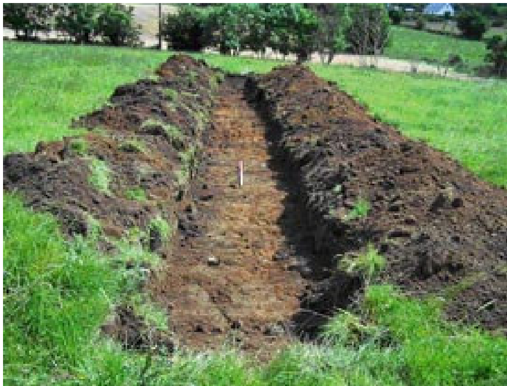
Plate Nine: Trench Four following excavation to the surface of the subsoil (Context No. 403), looking east.
