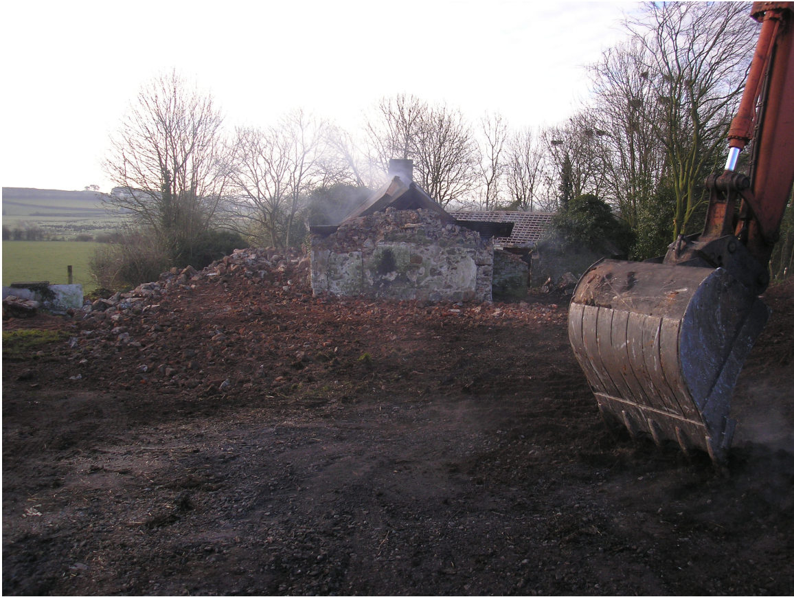
Plate 1: Application site prior to the excavation, looking south.
