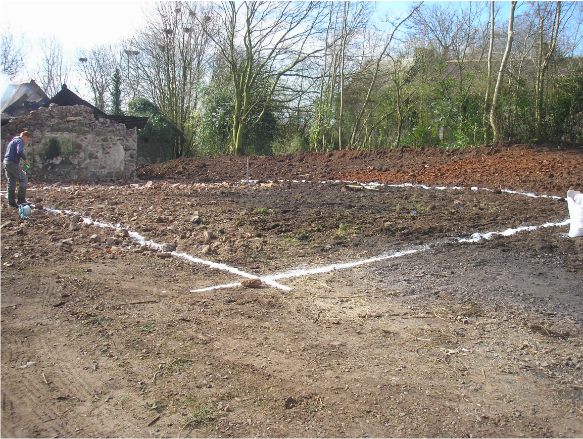
Plate 2: Layout of the foundation trench prior to the excavation, looking south-west.
