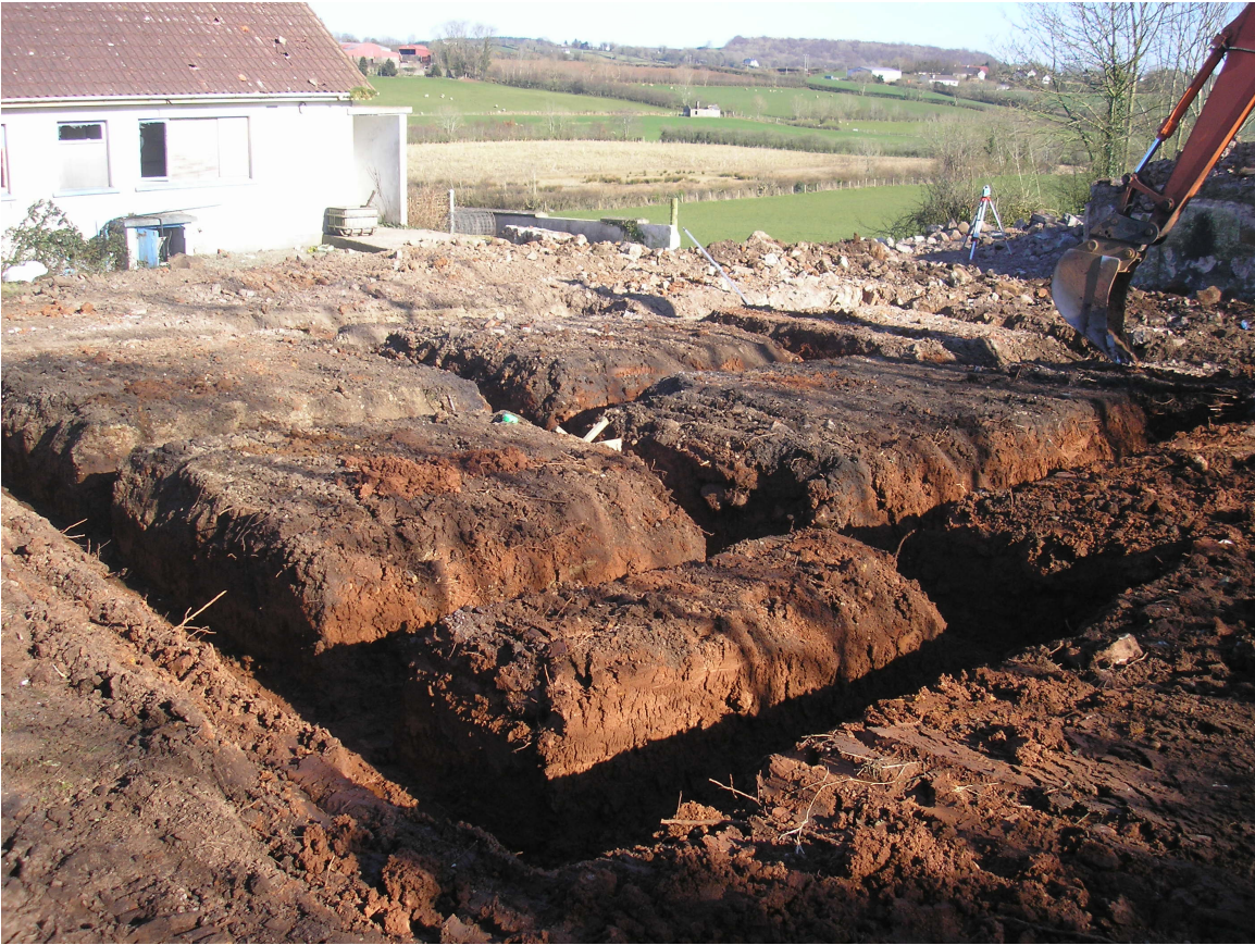
Plate 6: Application site following excavation of the foundation trenches, looking south-east.
