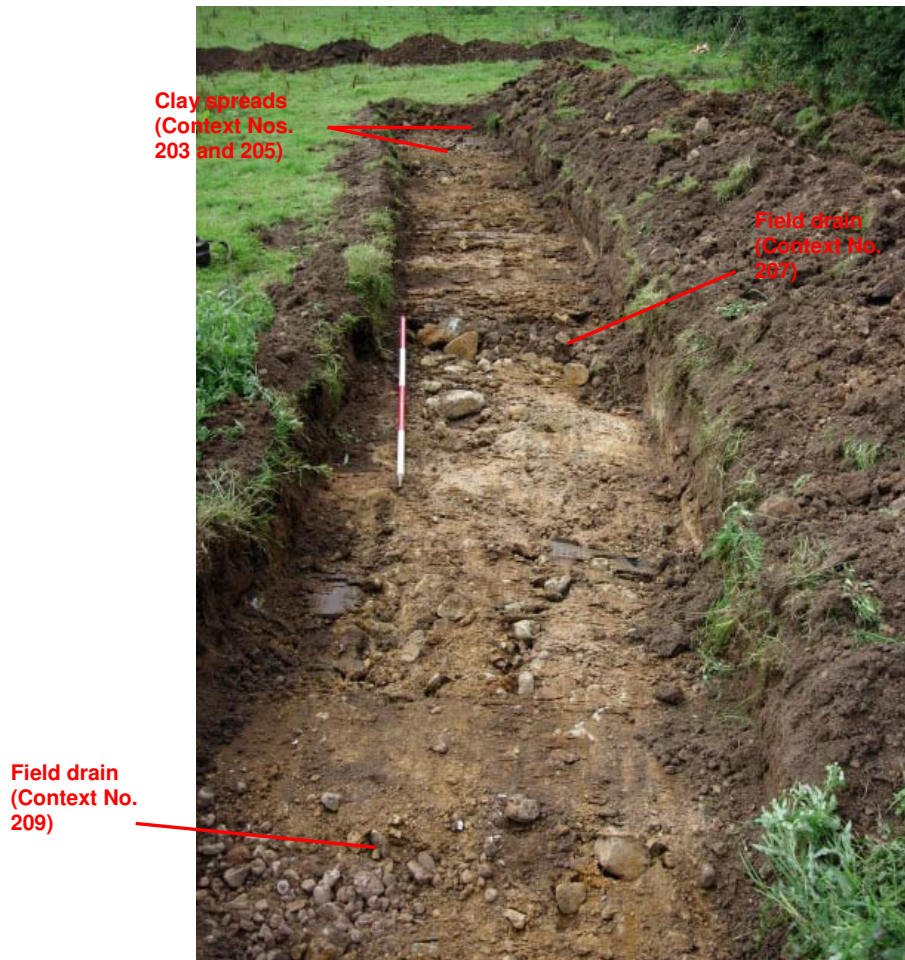
Plate Ten: Trench Two following excavation to subsoil (Context No. 211), looking west
