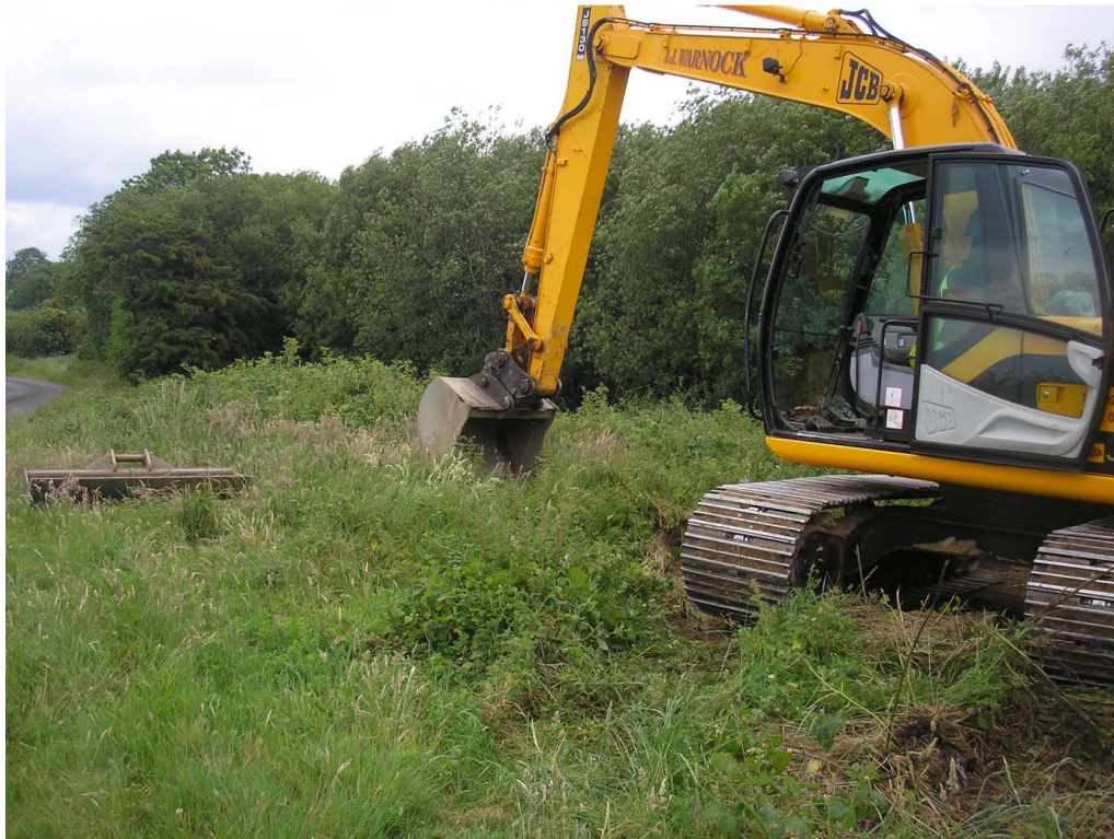
Plate Two: Application site prior to evaluation, looking north-west
