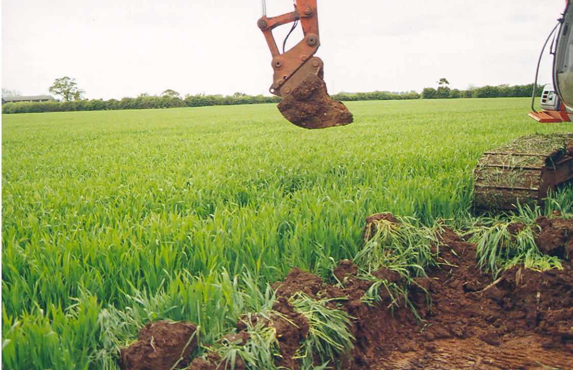
Photo 1: Excavation of Trench showing utilization of toothless “sheugh” bucket.
