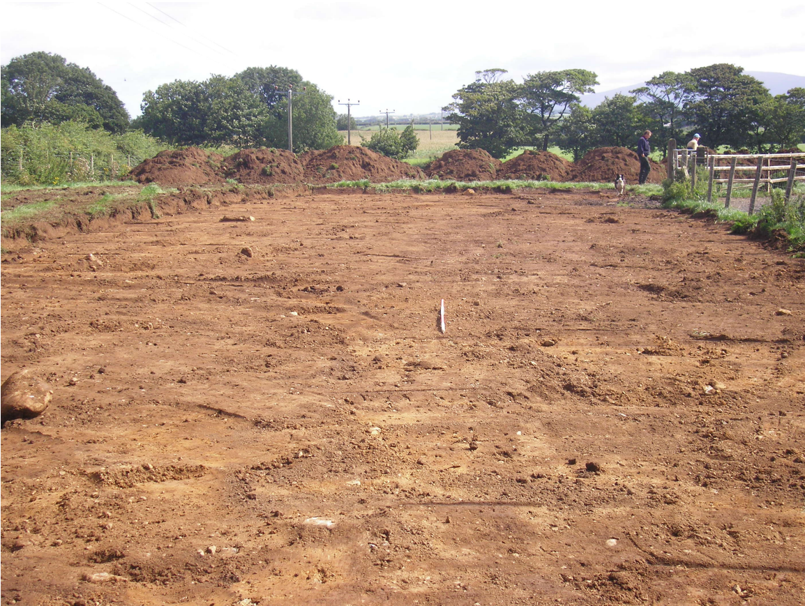
Plate 2: Following excavation to subsoil (Context No. 103) looking east
