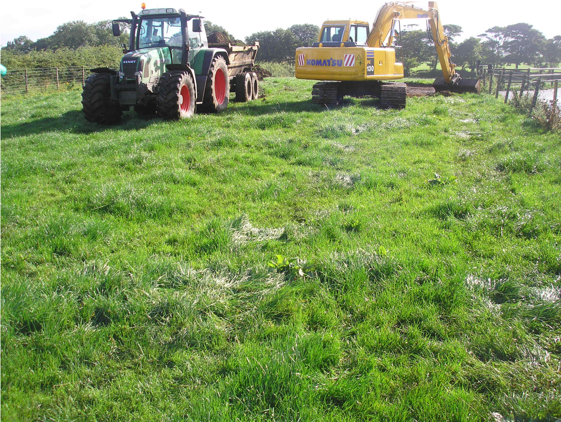
Plate 1: View of site before excavation looking east
