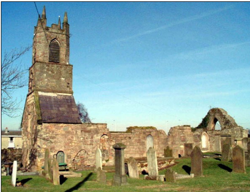
Plate Two: Hollywood Priory Church looking north – the top of the tower is a later addition.
