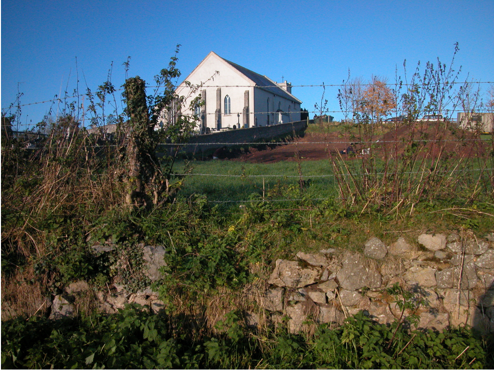
Plate C: Revetment wall looking east towards site and church
